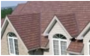
Roofing Contractors Palm Beach
