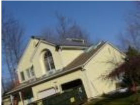
Chittenden Builders Roofing Contractors
