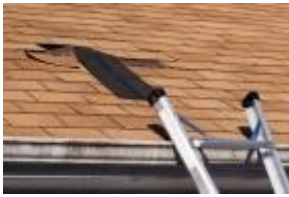
Roof Under Repair
