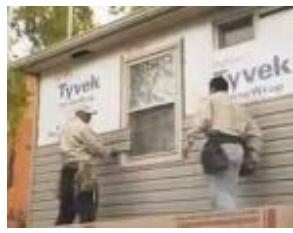
Home Siding Project
