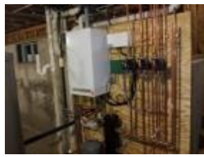
Furnace Repair Services
