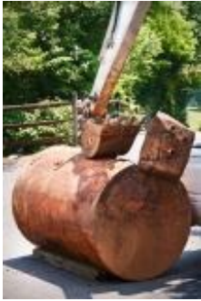
Underground Oil Tank Removal MA
