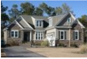
Wilmington Roofing Contractors
