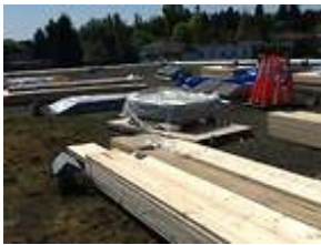
Commercial Roofing Project in Progress
